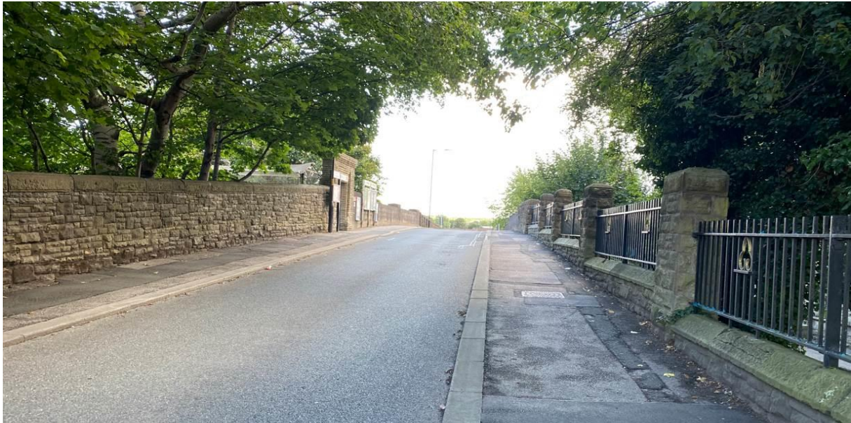
Figure 3 - Western approach, facing north east.
