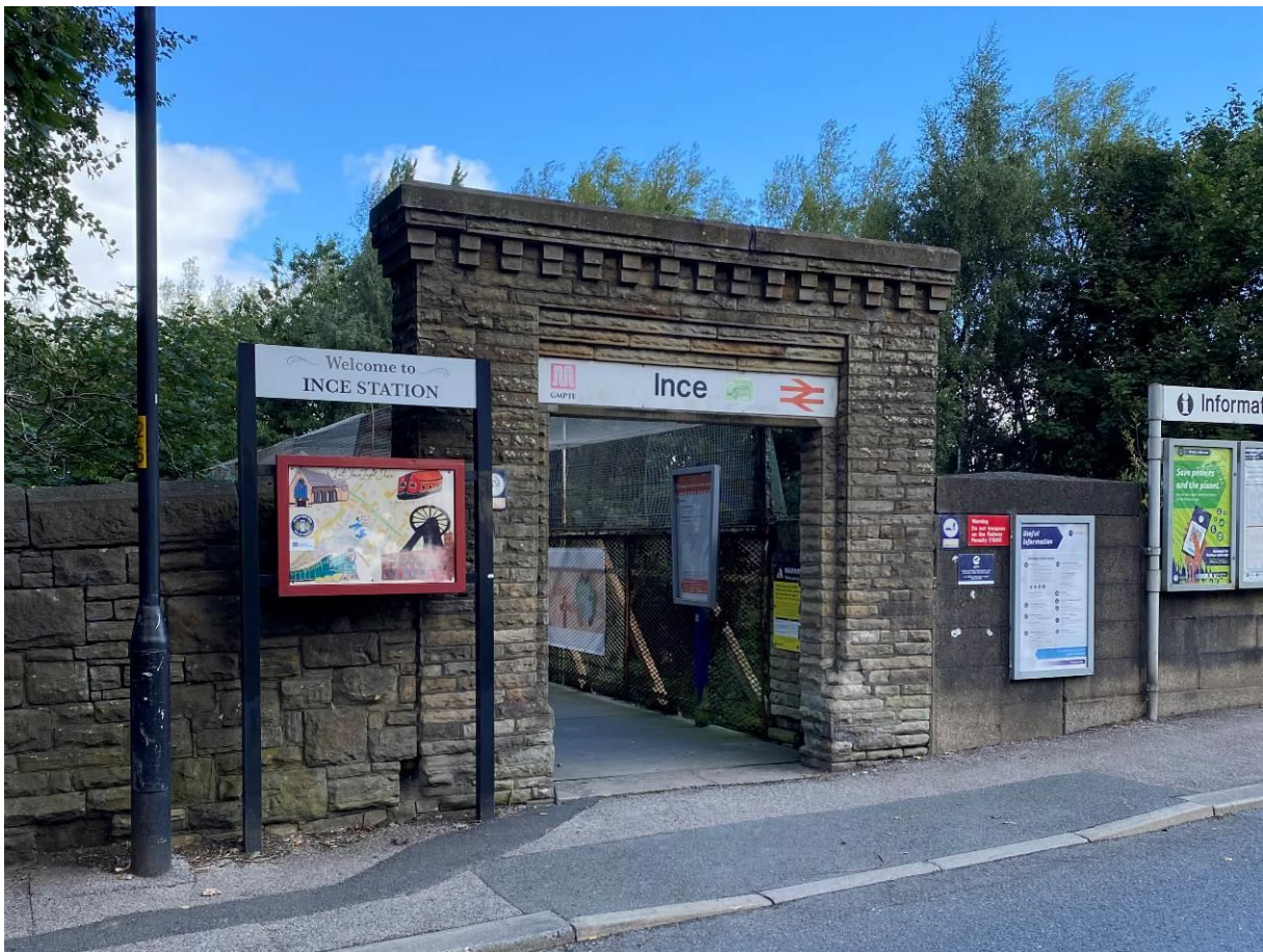
Figure 4 - The existing sandstone arch, denoting the entrance to the footbridge.
