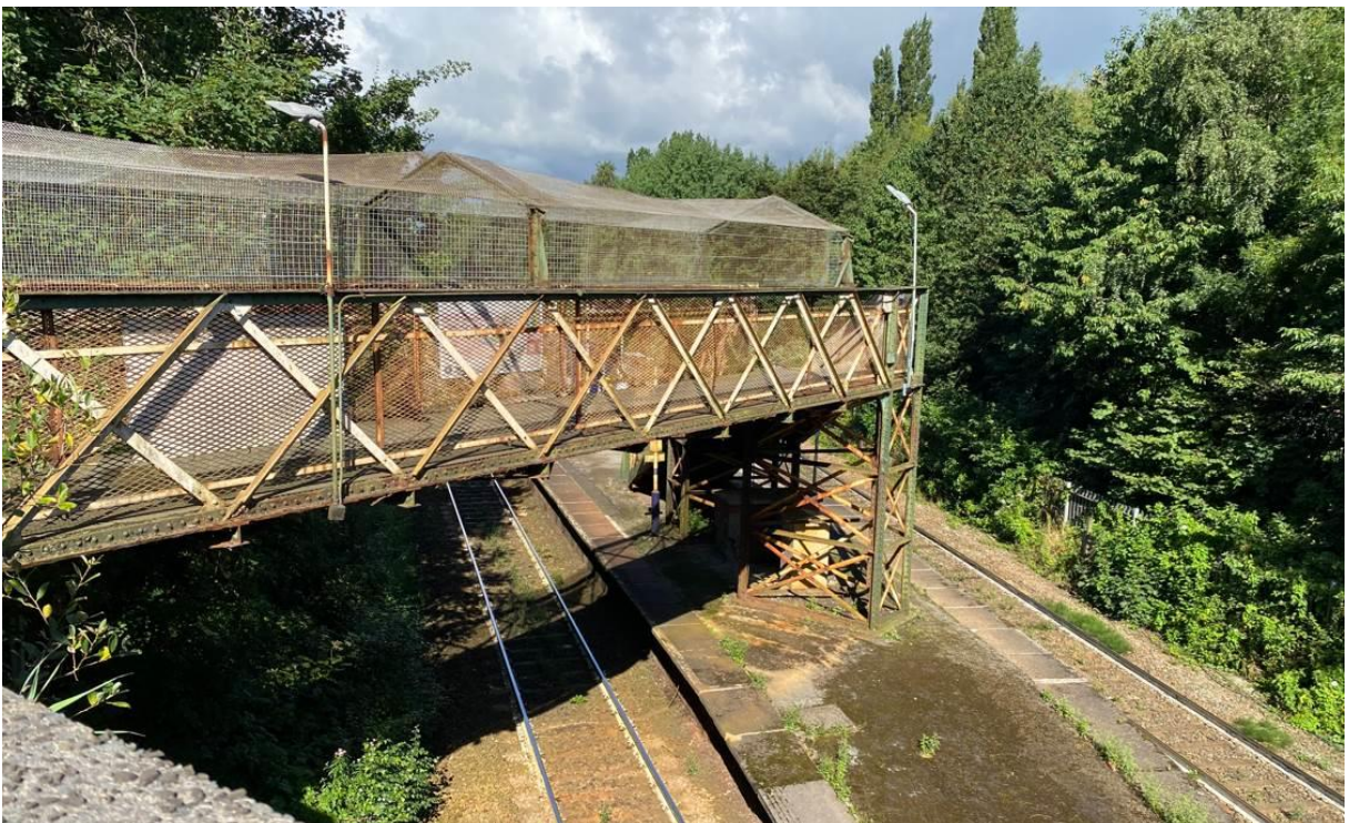
Figure 2 - View of footbridge from overbridge, facing west.
