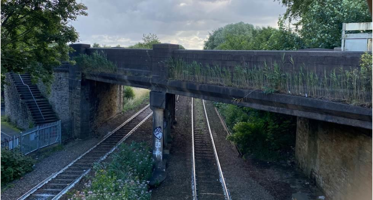
Figure 1 - View of overbridge from the pedestrian footbridge, facing east. The steps to Canal Street (to be decommissioned) can be seen to the left of the image.
