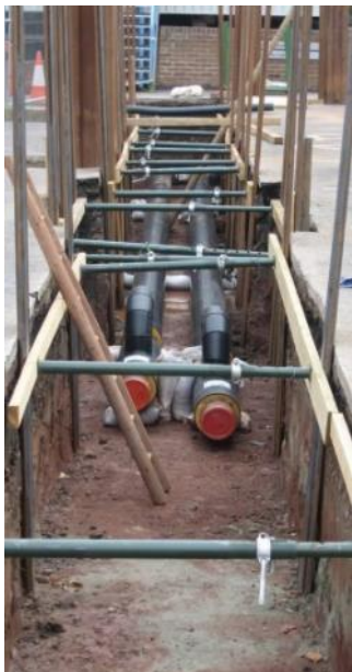
Figure 28 Ground Source Heat Pump Pipework
