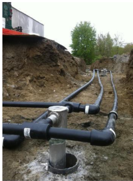
Figure 29 Ground Source Heat Pump Pipework Connecting to Boreholes
