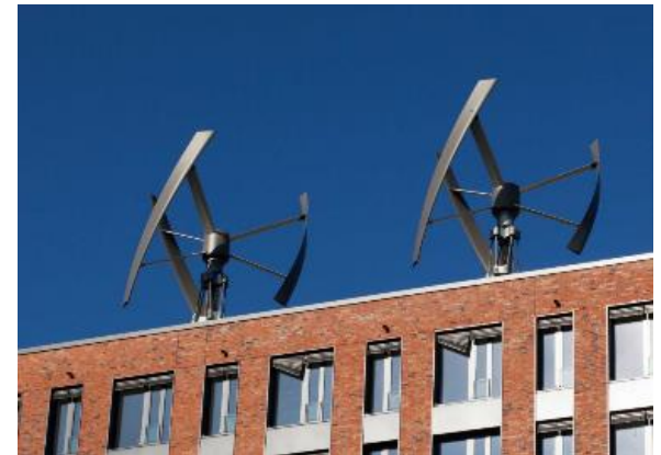
Figure 12 Typical Building Mounted Wind Turbine
