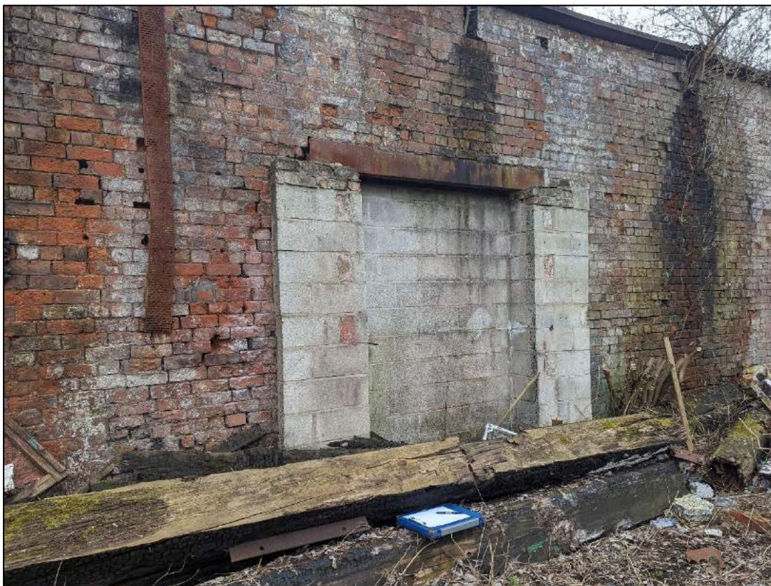
Plate 32: Detail of blocked loading door
