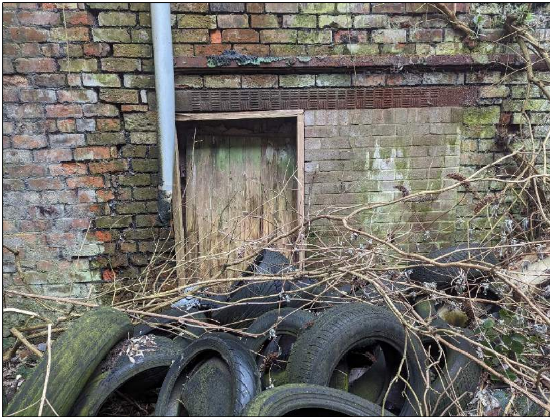
Plate 29: Detail of inserted and blocked loading doorway
