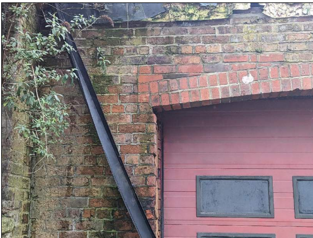
Plate 16: Detail of inserted lintel to loading door
