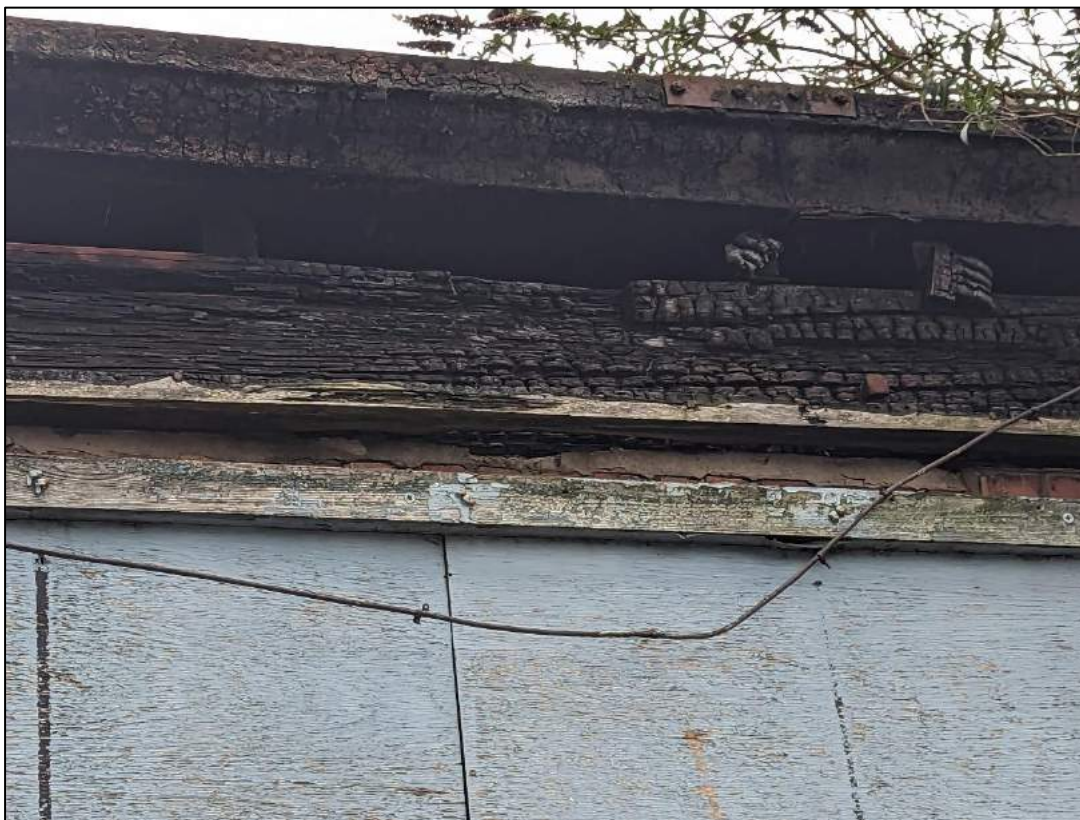
Plate 6: Fire damaged lintel to doorway
