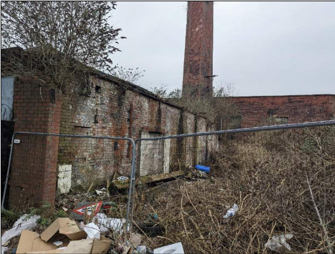
Plate 7: Collapsed elevation to central room to east of above
