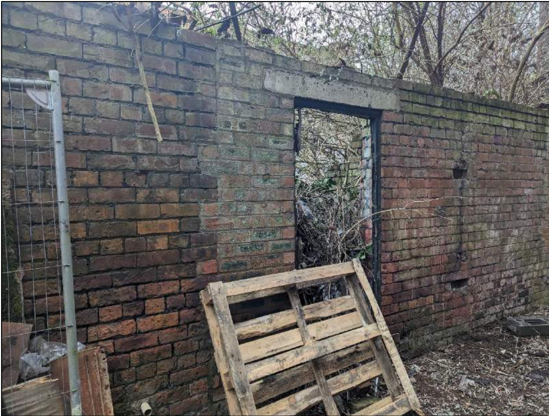
Plate 23: Detail of inserted doorway and rebuilt wall
