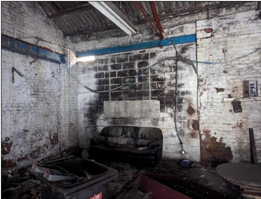
Plate 49: Blocked loading doorway in south end of west wall
