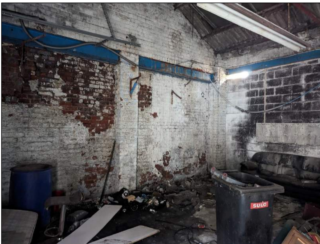
Plate 48: Blocked openings in south wall
