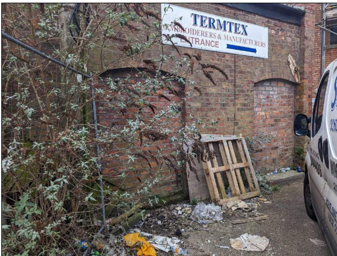
Plate 18: Blocked openings to north end of east elevation
