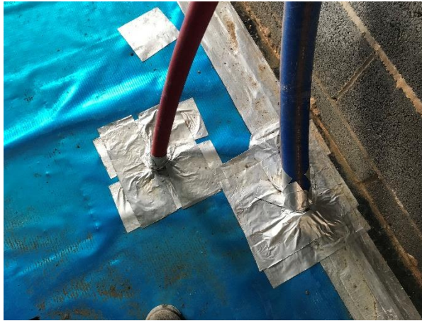
Figure 5 - Formation of top hat shapes using gas proof detail tape instead of using pre-formed top hats.
