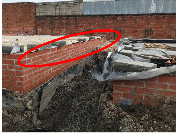
Figure 1 - Air bricks installed at <2m centres.
