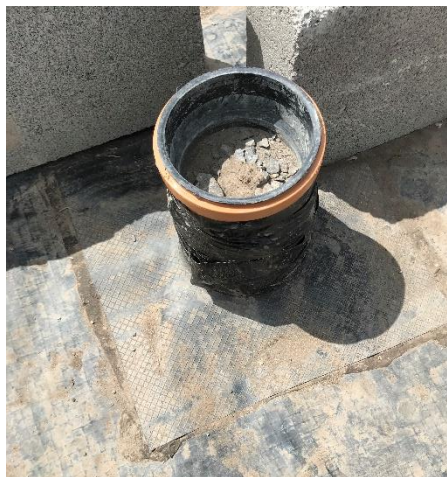
Figure 4 - Top hat installation with double-sided tape on all sides of top hat base and around inside of top hat sleeve. Jubilee clip around sleeve (under gaffer tape).
