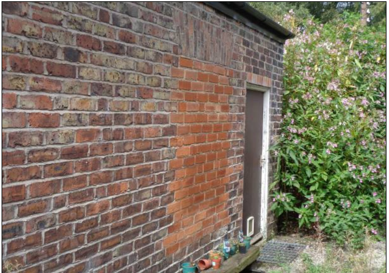
5. Blocked window and door at north end
